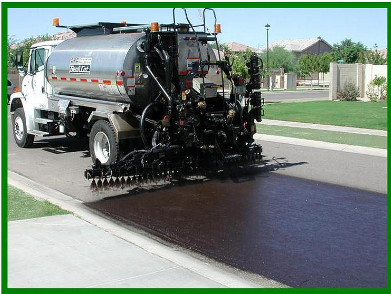
*Stone Lock* Fog Seal is a quick set light texture (QSLT) material consisting of a base, hard pen asphalt emulsion which is further prepared for resistance to environmental & chemical destruction through the interfusing of NEOS™ bio-resin modified ground tire rubber. Upon application the *Stone Lock* Fog Seal penetrates deep into tiny fissures and asphalt voids rejuvenating and flexibilizing the uppermost region of aged and embrittled asphalt.
